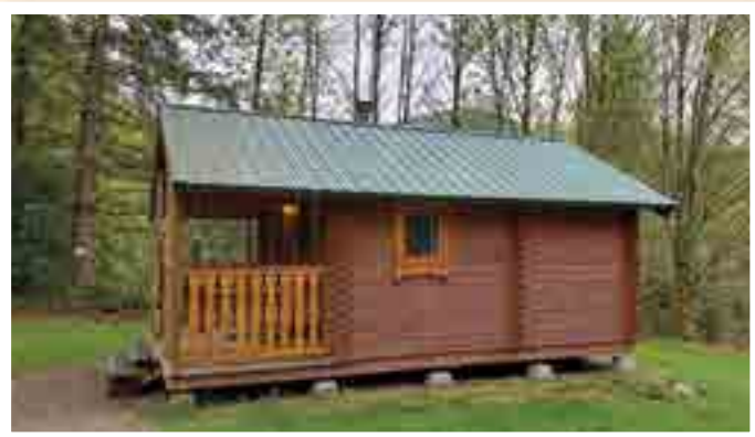
One of the Jim Creek's many cabins that were stained and cleaned during the closure.
